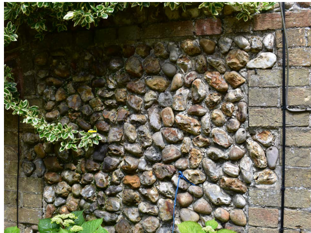
Figure 41: Clunch stone on boundary wall with brick border.
