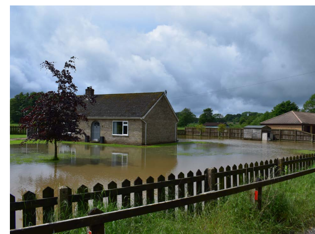
Figure 72: Example of flooding issues in Shouldham Parish.
