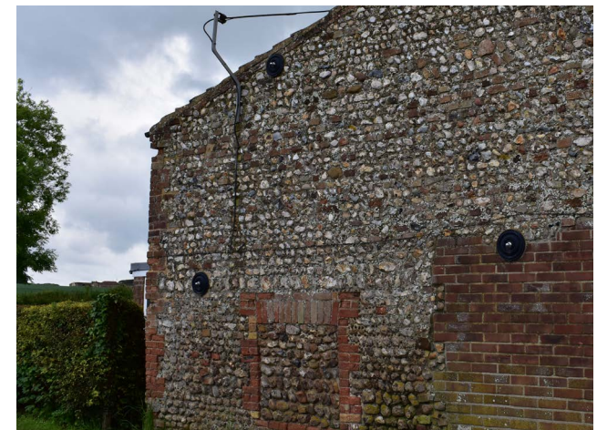
Figure 53: Example of a gable end displaying a mix of vernacular materials such as clunch and red brick.
