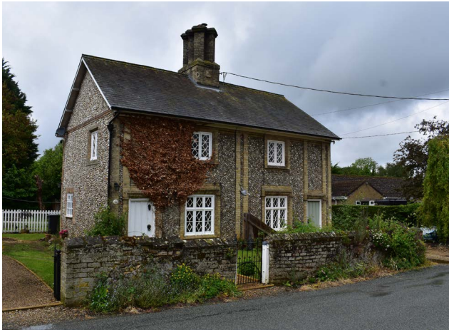
Figure 48: Alexandra Cottages, grade II listed.
