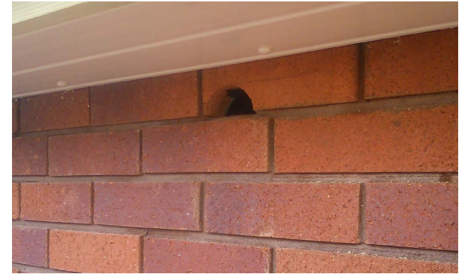
Figure 69: Example of a Swift brick under an eave.
