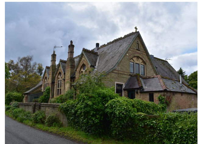
Figure 13: Former National School and Boundary Wall.
