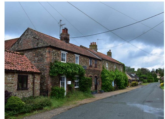
Figure 06: Row of terraced cottages on Westgate Street.
