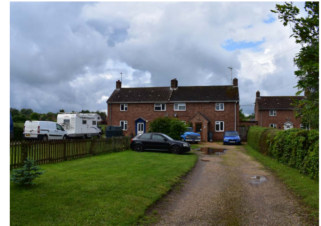
Figure 17: Semi-detached dwellings set back from the road on Eastgate Street.
