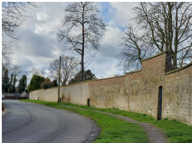
Figure 29: View 12A - From Eastgate Street by Victoria Hall's Drive entrance, to show wall.
