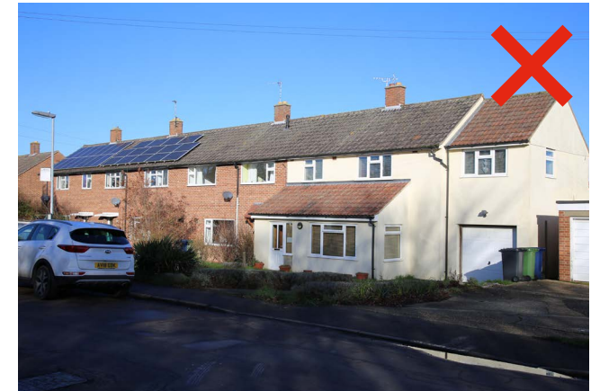
Figure 57: Negative example of a front extension which disrupts the existing building line and creates a substantial loss of front garden space and therefore contributes to surface water runoff.
